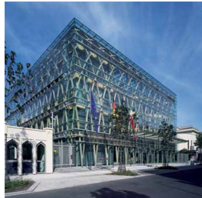
پروژه North Rhine-Westphalia ,State House of Representatives آرشیتهکت : Petzinka Pink
